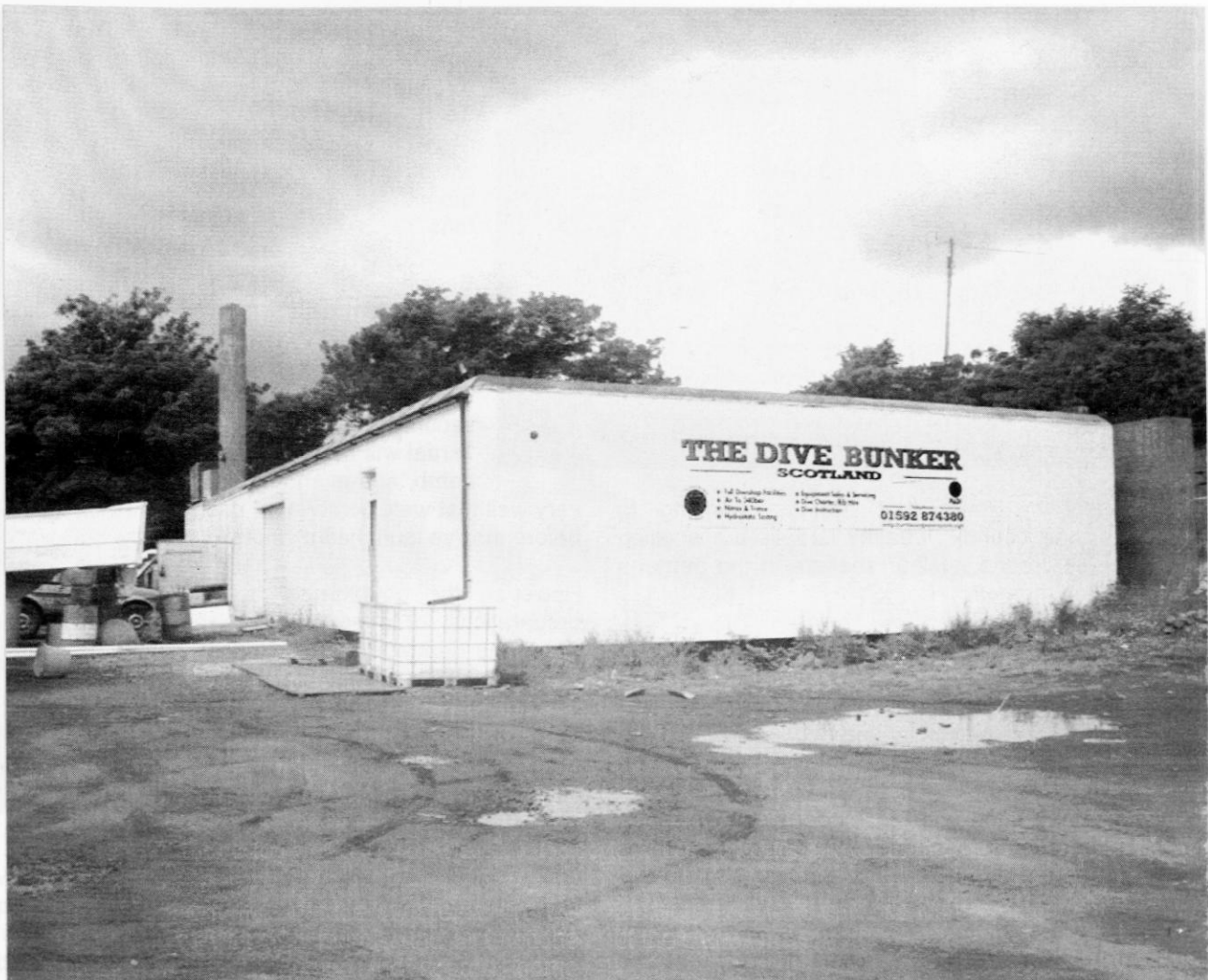
The 1950's emergency railway control centre at Burnisland built to replace Scotland Street - Photo by Nick Catford
